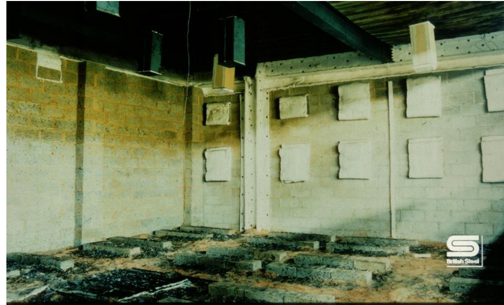
Floor deformation after the test
