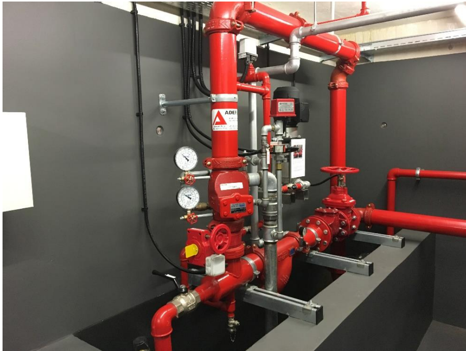
Underwater installation (normal)
